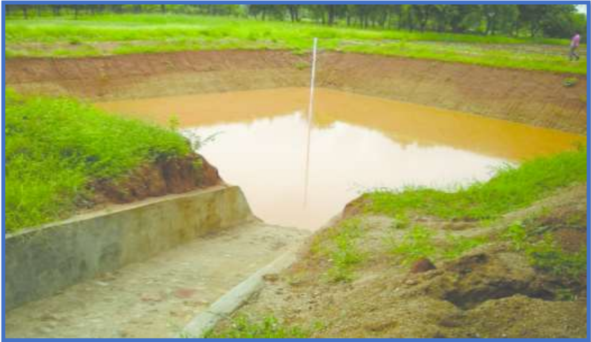
Typical farm pond with runway
